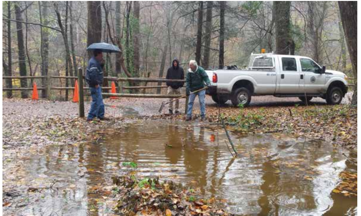
Heavy rain washed out the Pachella Field gravel access road onto Forbidden Drive last year.
