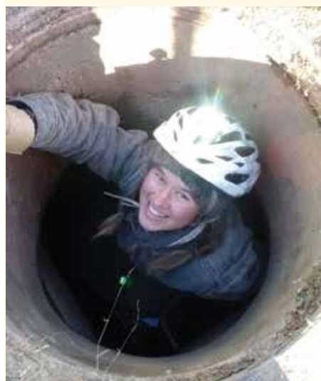
What lurks beneath is the farm's water system shutoff valve.
